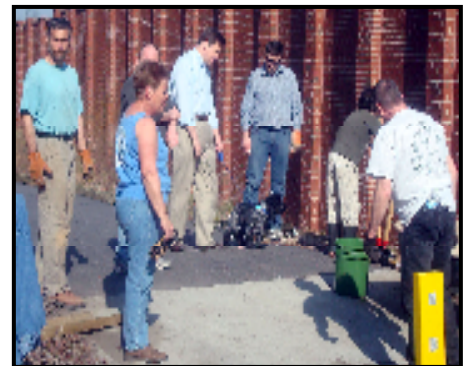
Volunteers work on the Brookline Trail
